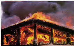
Conventional fireproofing may limit damage in case of fire, but it can also lead to roof rot, costing Americans an estimated $2 billion a year in repairs.
