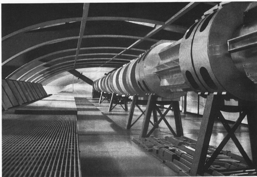
Horizontal intermix chamber (looking aft)
