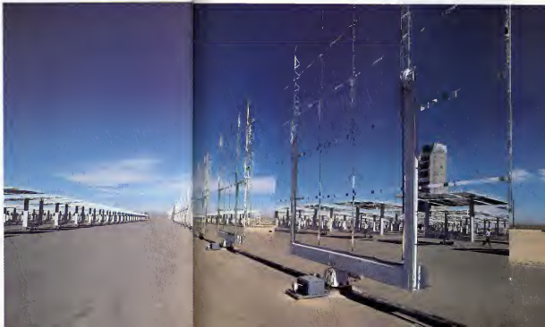
Sandra Lutzowsky a mirrored heliohelio reflect and focus New Mexico sunlight onto Power tower to generate electricity
